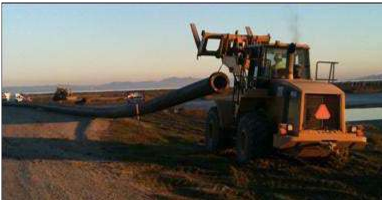
Figure 11 Typical beach-placement operation for sand pumped from a nearshore vessel.
