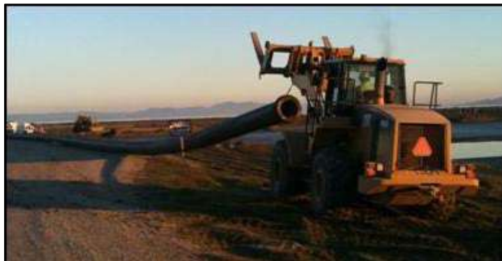
Figure 9. Typical beach-placement operation for sand pumped from a nearshore vessel.
